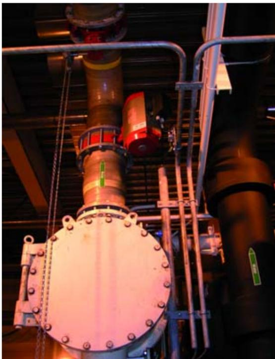
Picture 2: Position of cast-iron valve compared to duplex SS seawater cooler.
